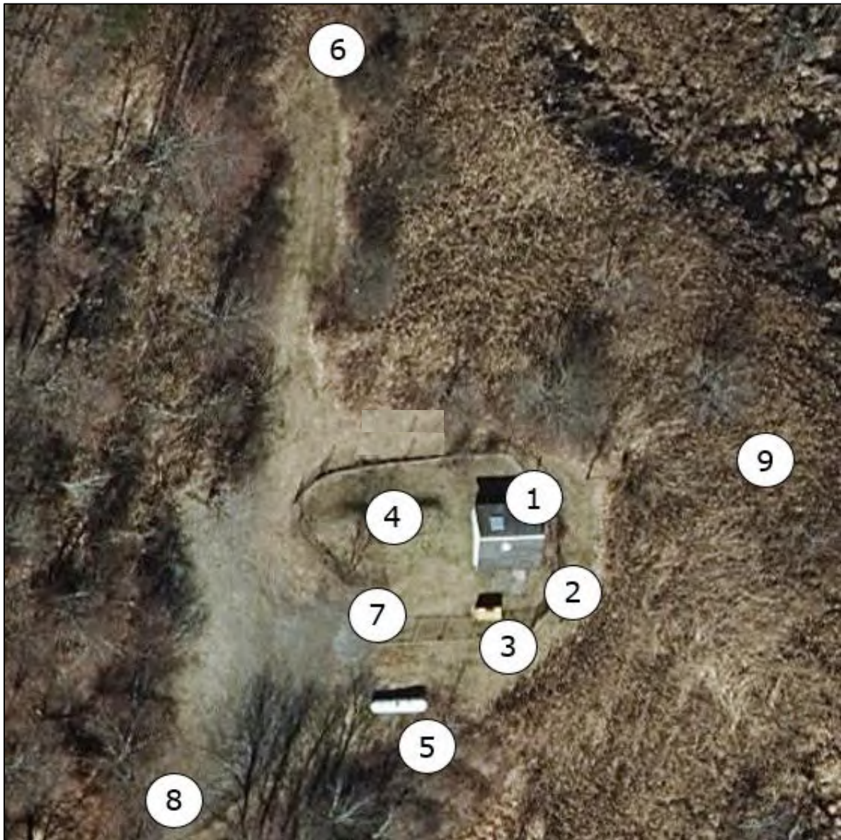
FIGURE 1-8 Quaker Hill Water Treatment Facilities
