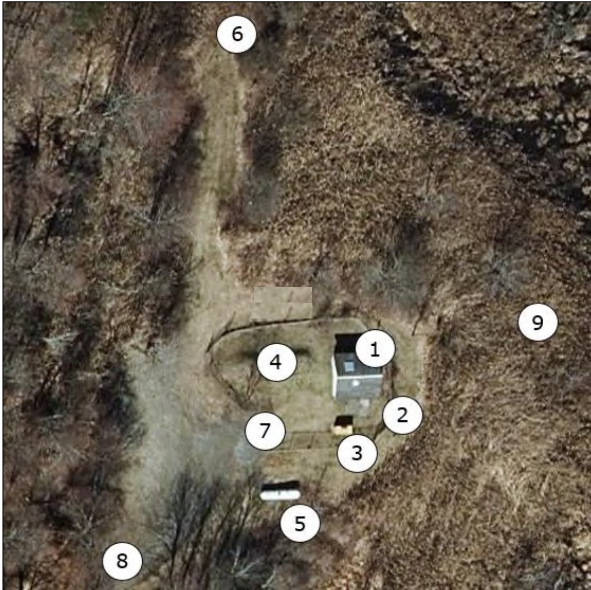
FIGURE 1-8 Quaker Hill Water Treatment Facilities
