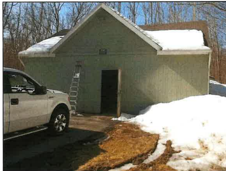
Figure 2-4 Pinebrook Treatment Facility
