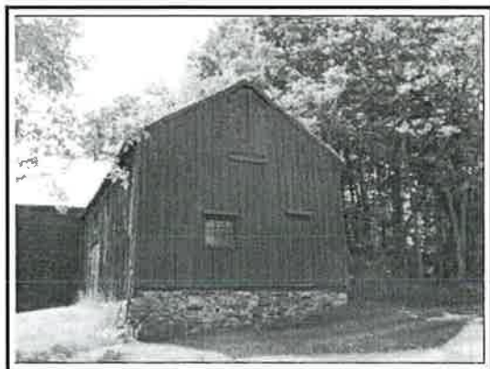
E end of Old Dairy Barn
